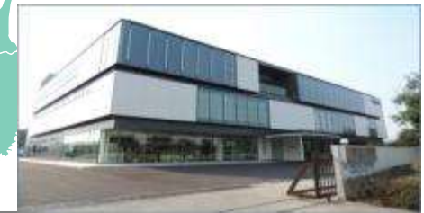
Haga T/C (Completed in Nov 2013)
