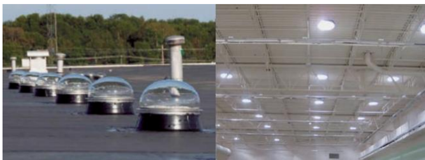
F&PA using natural light by light pipes
