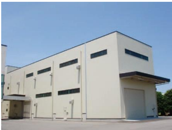
New technical building restored in FY2011
