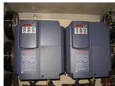
Inverter units for paint pump
