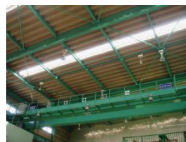
New skylight in the press area
