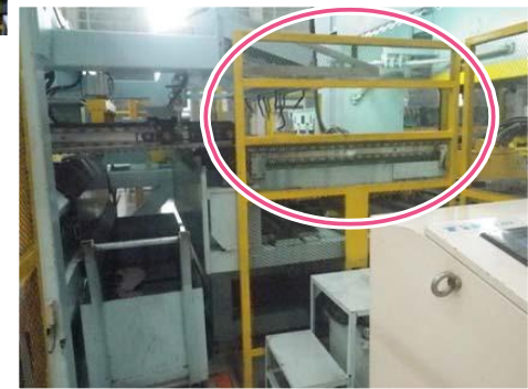
After: the height of safety fence built up higher. (1800mm standard)
