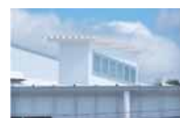
Installation of natural daylight intake window
