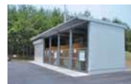
Garbage Station completed
