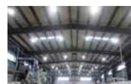
Shot/Finishing building completed
