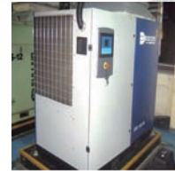
Introduced inverter type air compressor
