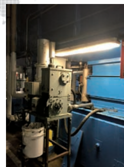
Installed magnetic filter in warm water washing process in the coating process
