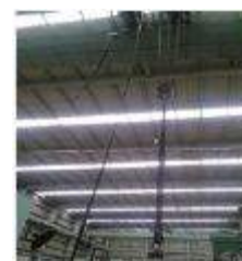
Warehouse and manufacturing area lighting
