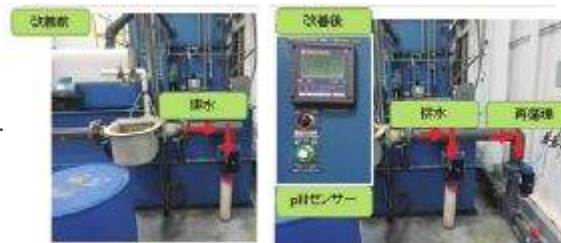
Improvement of pH level monitoring system
