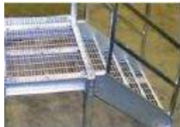
Stairs with anti-freezing measures
