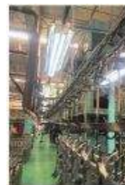
LED lighting installed in the factory
