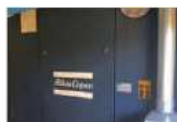
AtlasCopcoGA 315, 369 horsepower screw air compressor
