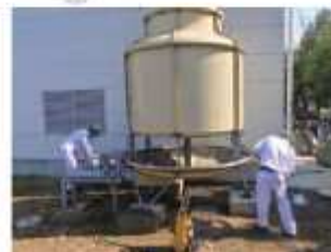
Regular maintenance and cleaning of the cooling tower
