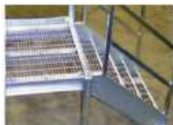
Stairs with anti-freezing measures
